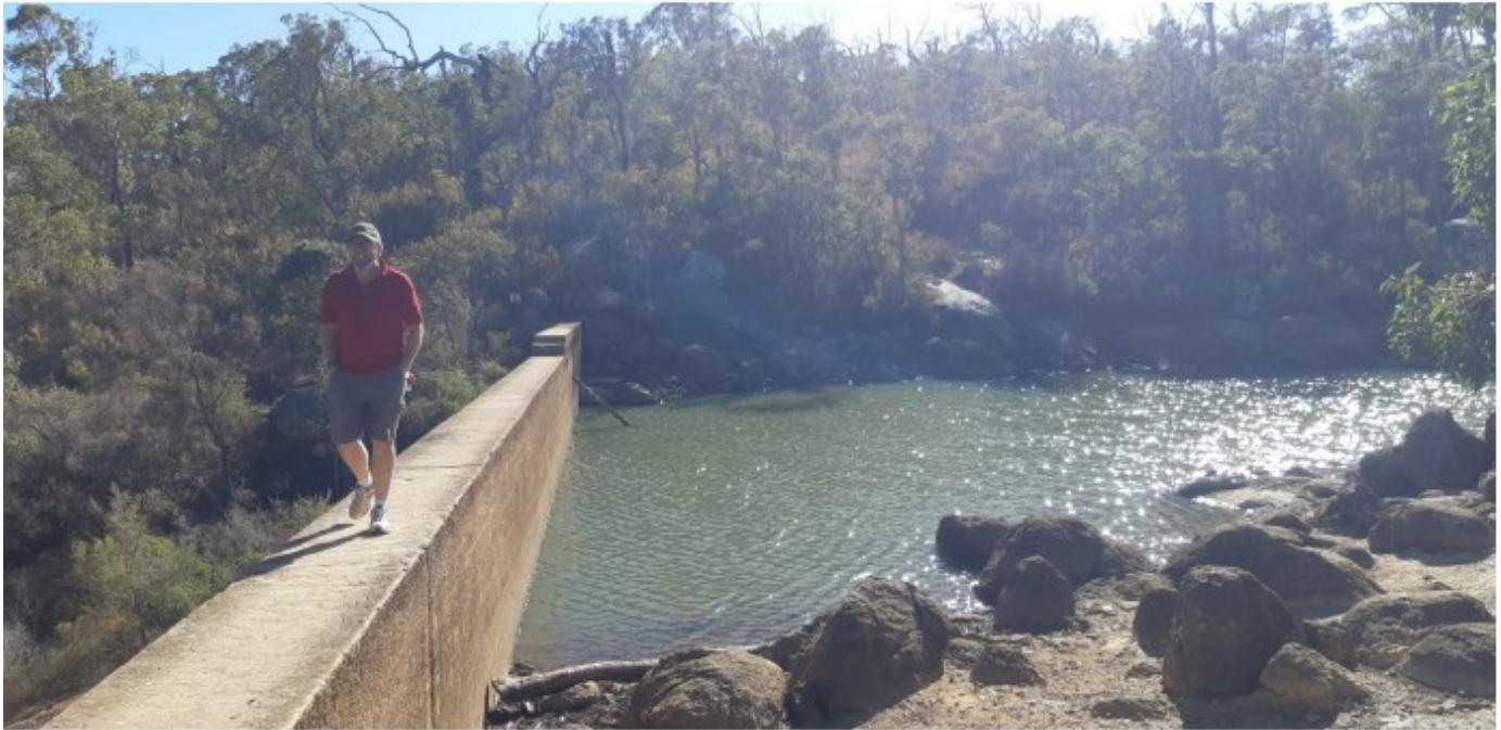
Brian walking the dam wall.
